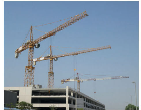
Potain cranes from NFT Specialised in Tower Cranes.
