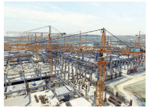
Istanbul New Airport has 58 Liebherr tower cranes.
