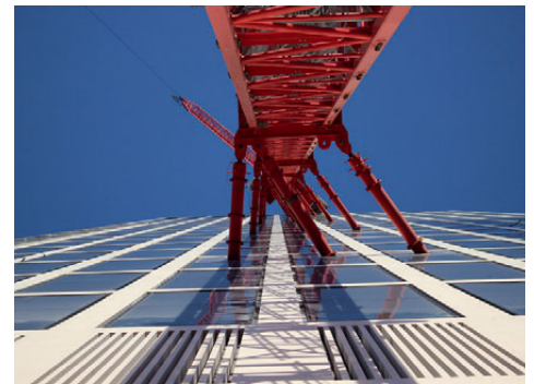
■ A view of the anchor system of a Wolffkran crane.
