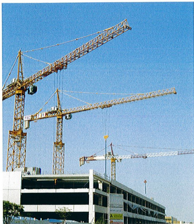
Potain hammerhead cranes are used to construct an Al Tayer Group showroom.
