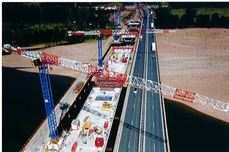
A series of Raimondi cranes are temporarily suspended over a river as part of a bridge expansion.
