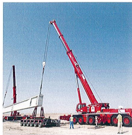
Tandem lift of concrete beam by Demag cranes.
