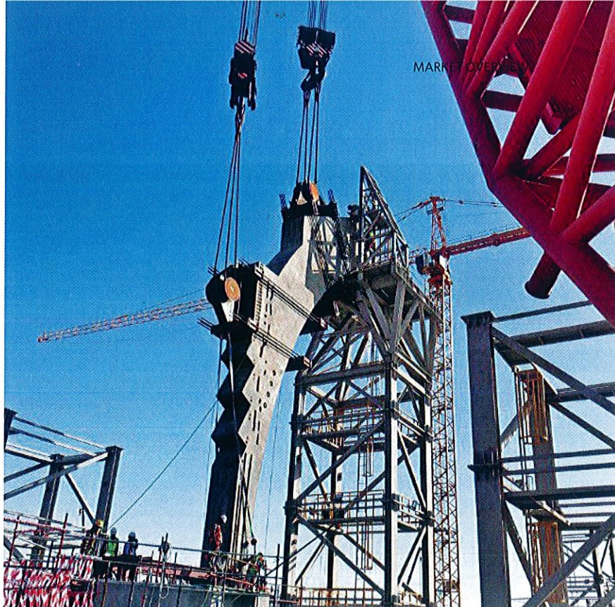
Mammoet crane installing precast sections of the new terminal at Kuwait International Airport.
