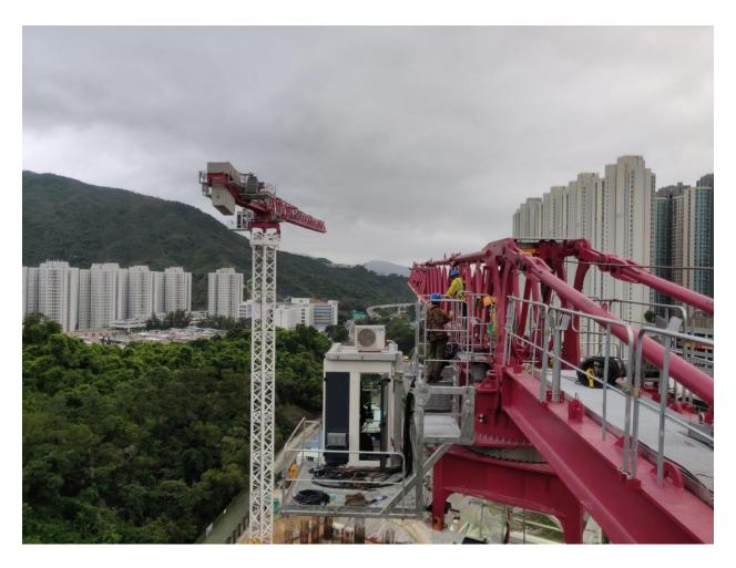
Two MCT 565 units, the largest topless Potain crane in the Asian market, and three MCT 385 units supplied for their ease of transportation and erection at the job-site.
