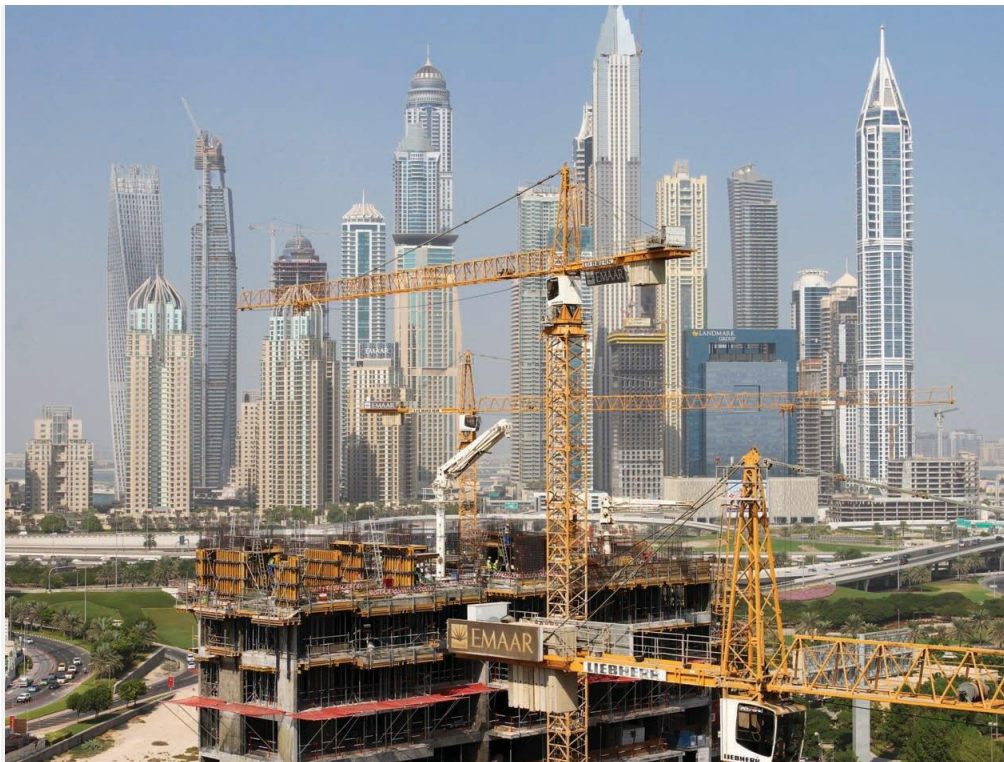
tower cranes building “The Hills”, a four-tower development in Dubai.
