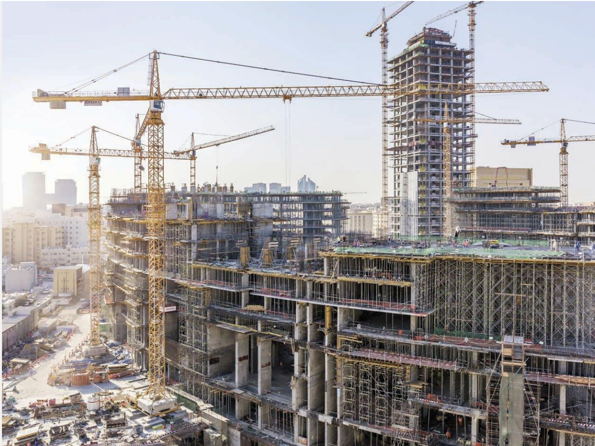
15 top slewing Liebherr tower cranes to Doha Oasis with hook heights between 53.5m and 169m
