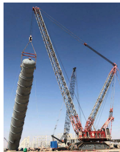
ALE using a CC8800-1 to lift a refinery component and a CC2800 as tailing crane at the Karbala Refinery, Iraq.
