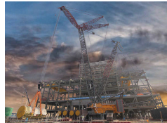
Al Faris used a Liebherr LR 11000 to lift a 404t generator for a Dubai power plant.
