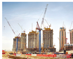
Raimondi LR213 luffing crane erected at Dubai Creek Harbor
