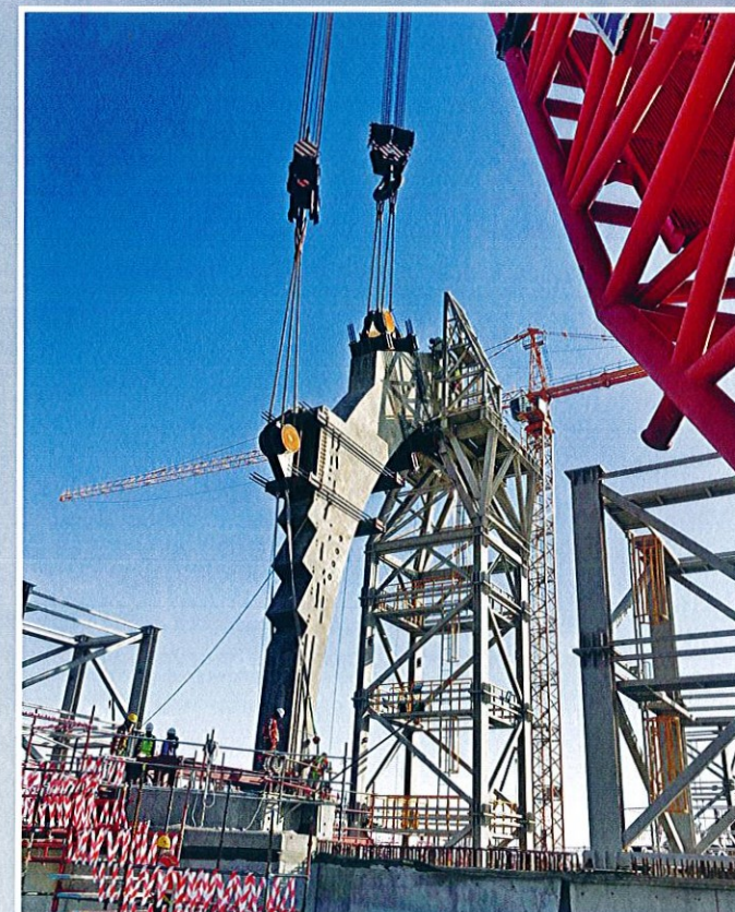
Mammoet installed this first precast concrete element, in a tandem lift using two 600t crawler cranes.
